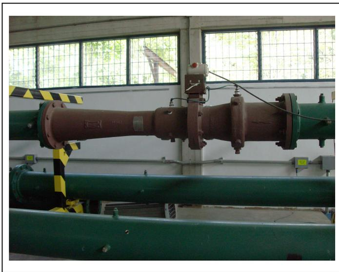
Figure 1. Venturi meter in a 10 inch pipeline
